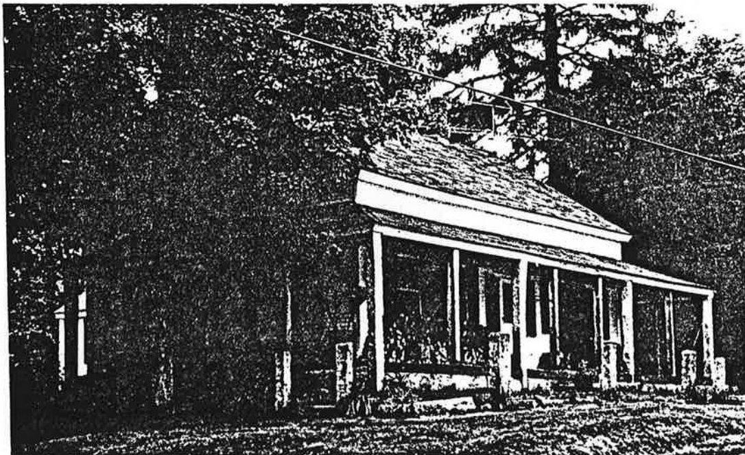
Across from the Union Church the Goodwin House features a unique porch supported by granite posts above a granite foundation.
